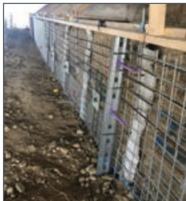
Underpass in VIC, using shotcrete stabilisation
