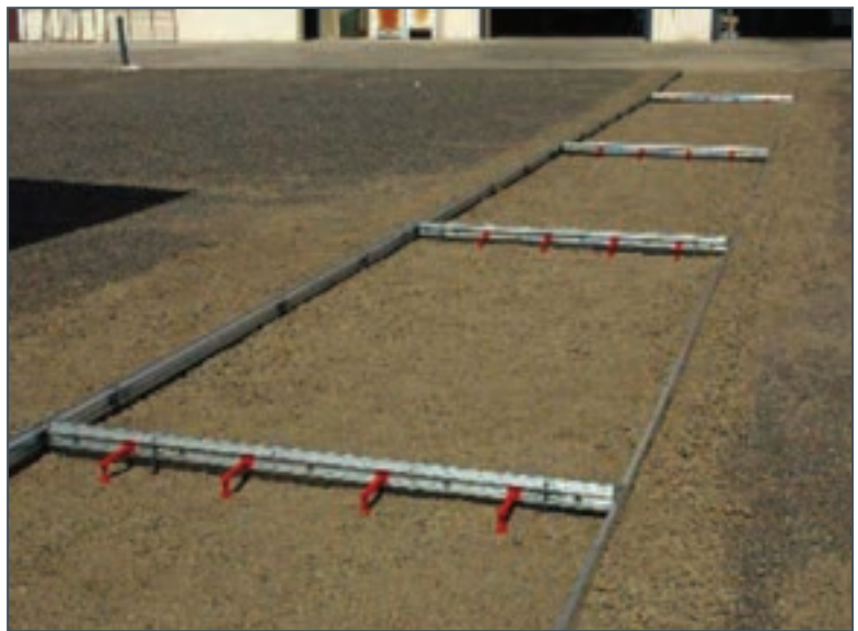
Connolly Expansion Joint System in use on a concrete footpath
