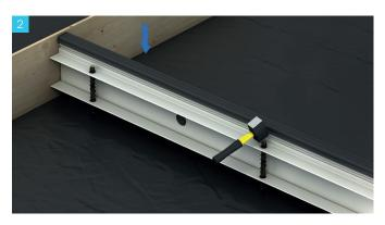
Position the expansion joint profile in the desired location and drive in the supplied pegs. Ensure the top of the peg is at least 20mm below the intended level of the finished concrete.
