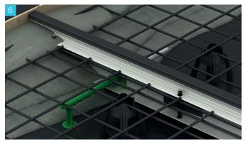
Place reinforcement and pour concrete evenly to both sides of the expansion joint at the same time. Finish surface and ensure top of joint is clear of any concrete.
